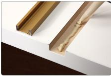
Cut a 1-1/8" wide x 1/2" deep groove in Apply a bead of heavy duty construction adhesive like Liquid Nails®.
