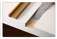
Use a putty knife or chisel to flatten the bead.
